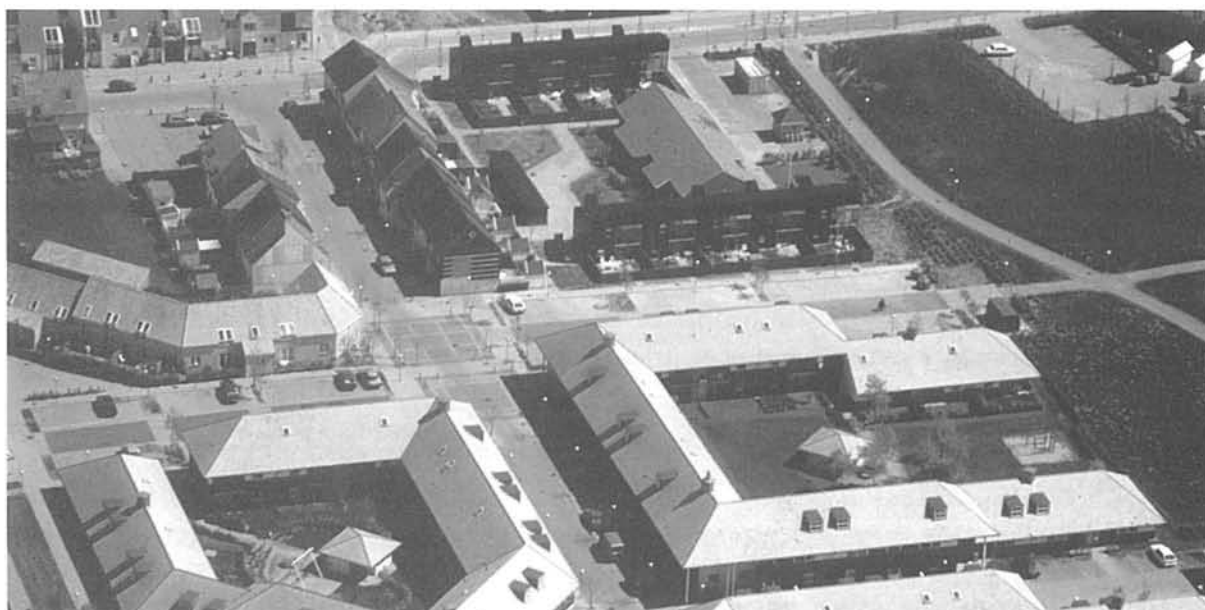
Fig 9. The planning of the housing area with a subdivision into well defined neighbourhoods was a main issue in the "code" estates shown in this photo from Egebjerggård
